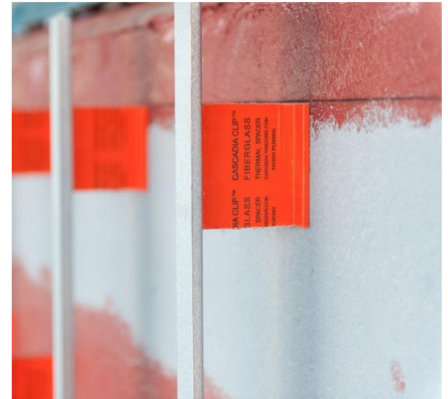
THERMAL SPACER FOR CLADDING SUPPORT SYSTEMS
