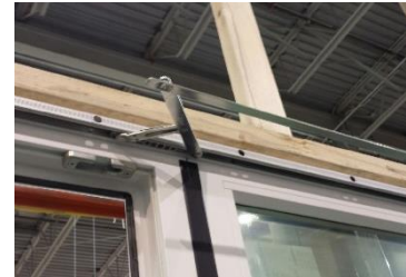
Figure 5: Scissor Gear Installation
