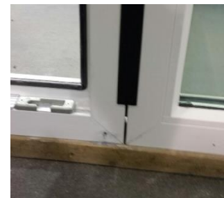
Figure 2: H-Bar Installation
