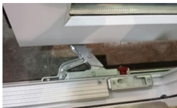
Figure 8: Bogie Installation Position
