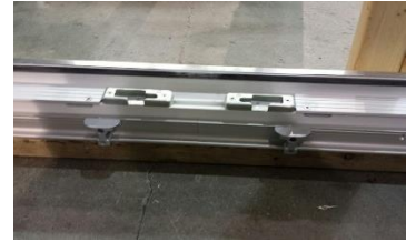
Figure 4: Sill Track Glider Location
