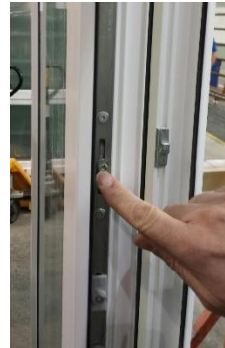
Figure 14: Gasket Tightness Adjustment
