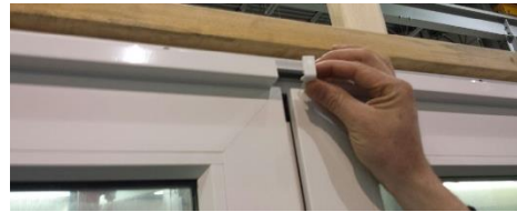
Figure 12: Sash Track Caps Installation
