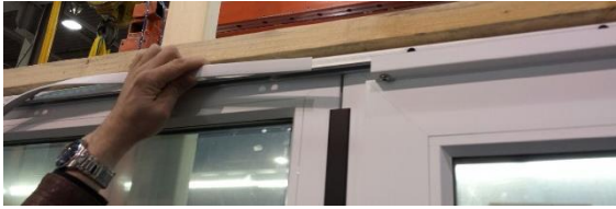
Figure 11: Sash Track Cover Strip Installation
