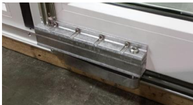
Figure 13: Vertical Sash Adjustment
