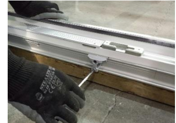
Figure 15: Sill Track Glider Adjustment
