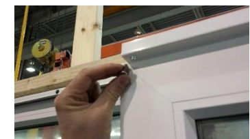
Figure 10: Securing Scissor Gear in Sash Track
