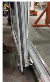
Figure 9: Sash Leaning 20° for Installation
