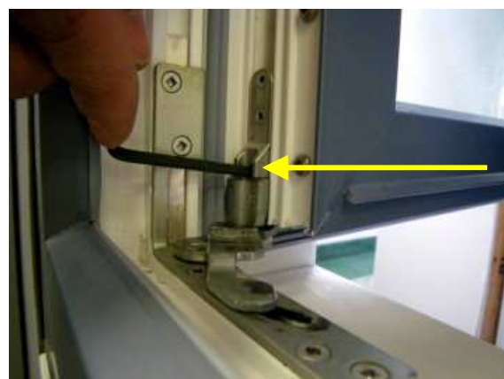
Figure 4 – Left/right adjustment (bottom of sash) Rotate wrench indicated at arrow for adjustment
