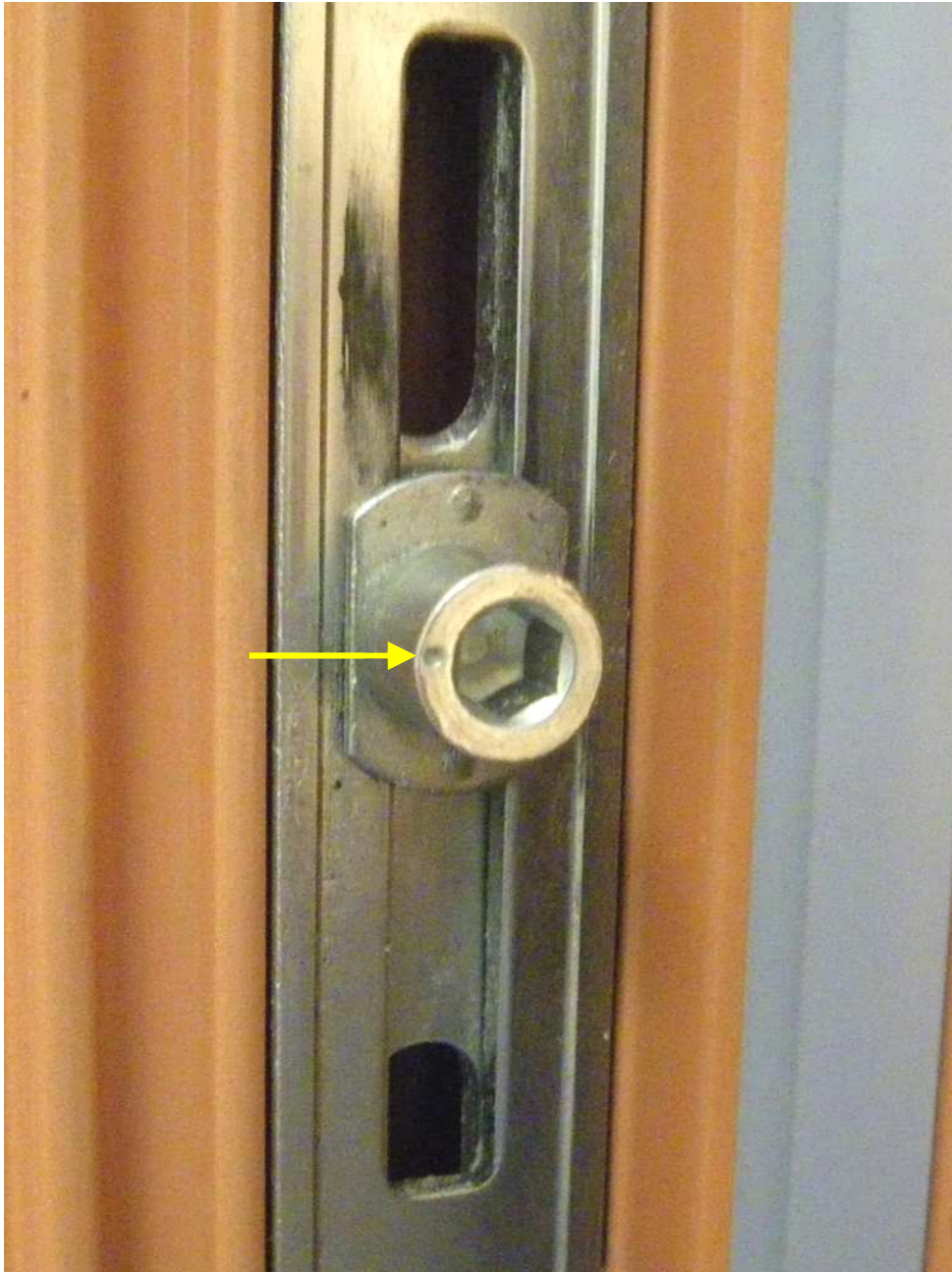
Figure 9 – Typical lock cam on multi-point hardware. Dot on left side of cam's perimeter is the adjustment indicator. Loosest setting: indicator dot is on exterior side of cam. Tightest setting: indicator dot is on interior side of cam. Middle setting: indicator is on top or bottom.
