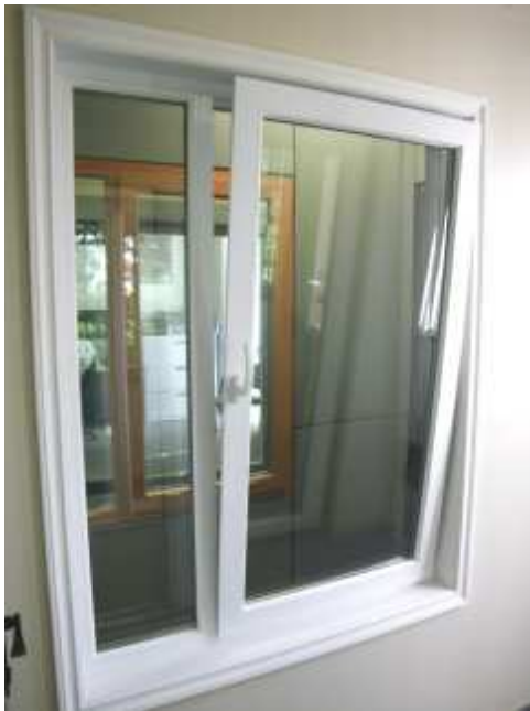
Window - Interior view
