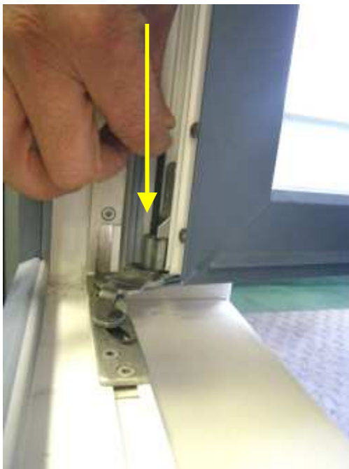
Figure 3 – Up/down adjustment (entire sash) Rotate wrench indicated at arrow for adjustment
