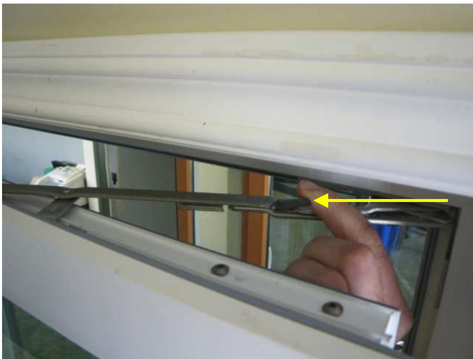
Figure 7 – Left/right adjustment (top of sash) Rotate wrench indicated at arrow for adjustment
