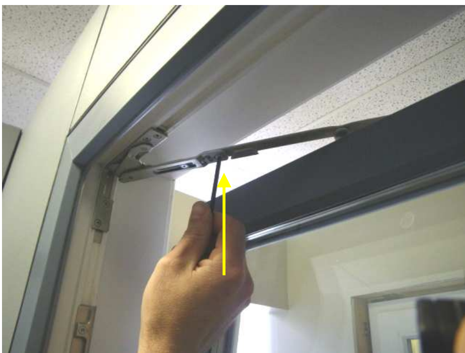
Figure 8 – Inward/outward adjustment (gasket compression at head of sash) Rotate wrench indicated at arrow for adjustment
