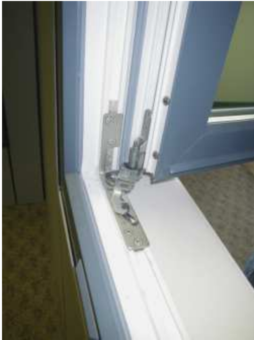
Figure 1 – Bottom hinge at window (window open, turn function, viewed from exterior)
