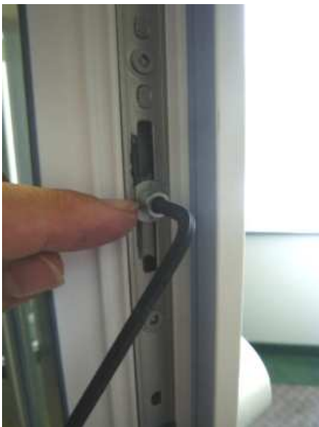
Figure 10 – Inward/outward adjustment (gasket compression at lock cam) Rotate wrench in lock cam for adjustment
