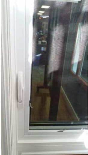
Window corner shown with screen installed Interior view
