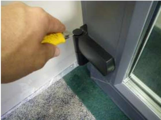
Figure 6 – Remove cap at top with flat tool
