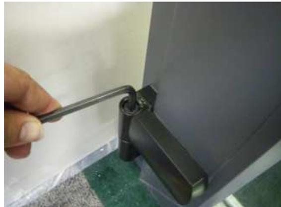
Figure 7 – Rotate Allen wrench for adjustment
