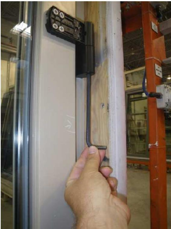
Figure 5 – Rotate Allen wrench for adjustment
