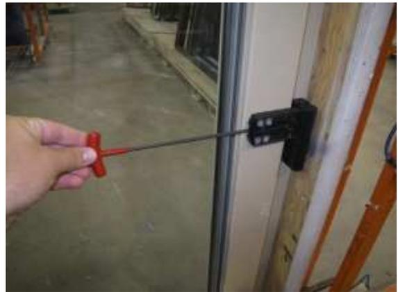
Figure 4 – Rotate Allen wrench for adjustment
