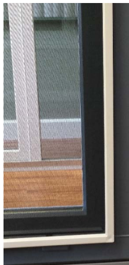
Window corner shown with screen installed exterior view
