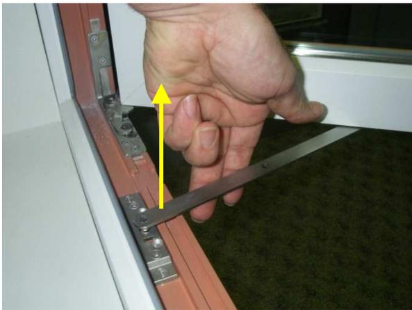
Figure 1 – Restrictor arm: pull to disconnect
