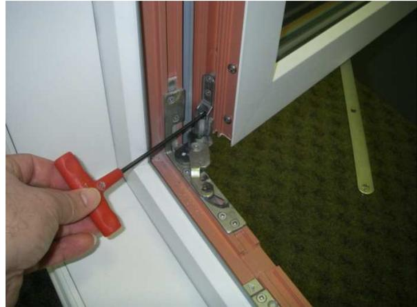
Figure 4 – Bottom hinge adjustment point (left/right)
