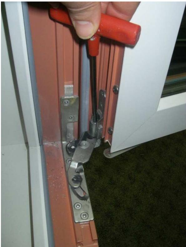
Figure 5 – Bottom hinge adjustment point (up/down)
