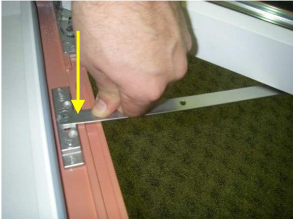
Figure 3 – Restrictor arm: push to reconnect.
