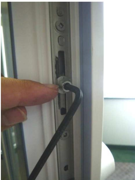
Figure 6 – Inward/outward adjustment (gasket compression at lock cam)
