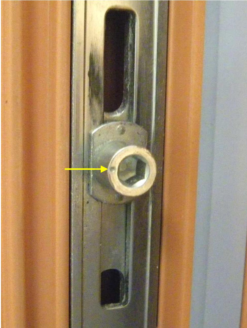
Figure 7 – Typical lock cam on multi-point hardware. Dot on left side of cam's perimeter is the adjustment indicator. Loosest setting: indicator dot is on exterior side of cam. Tightest setting: indicator dot is on interior side of cam. Middle setting: indicator is on top or bottom.
