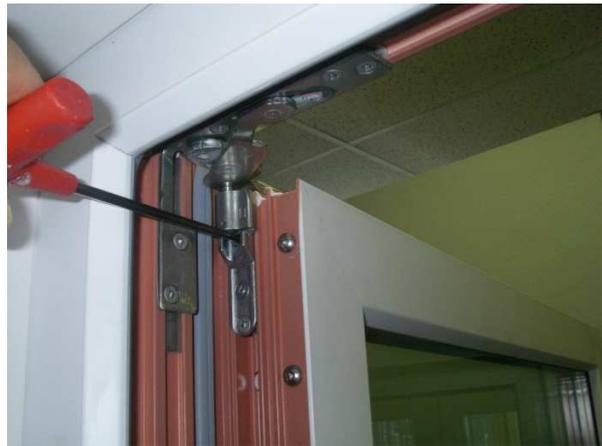
Figure 2 – Top hinge adjustment point (left/right)
